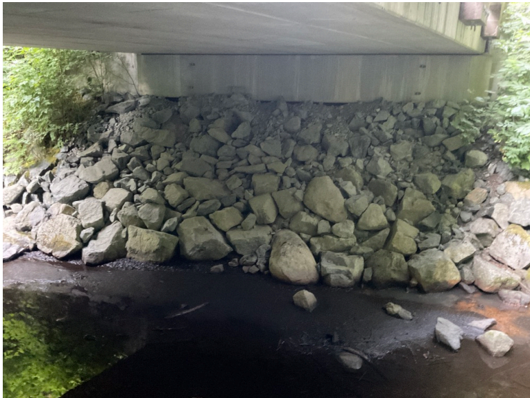
Right Bank Abutment when facing downstream
