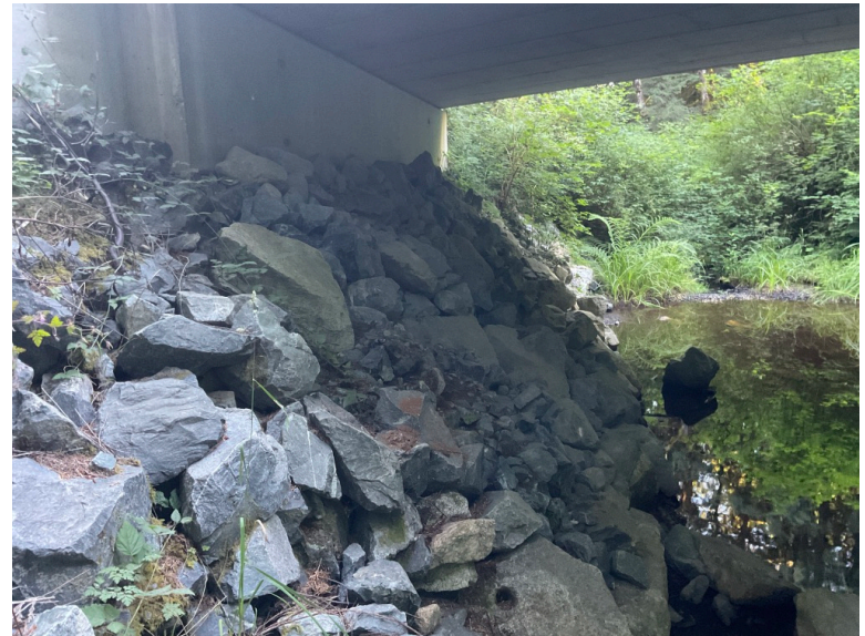
Left Bank Abutment when facing downstream
